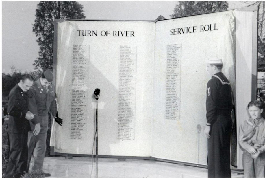
Turn of River Service Roll – located on the north side of Vine Road, near the entrance to the Wormser Senior Residence (formerly Willard Elementary School).
